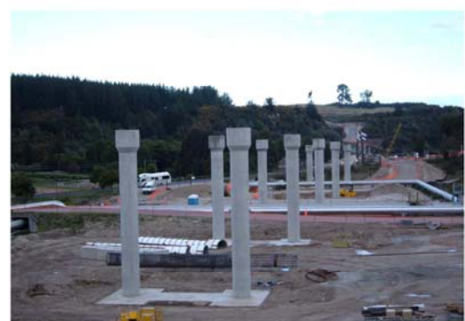
Contact Energy steam field flyover piers
