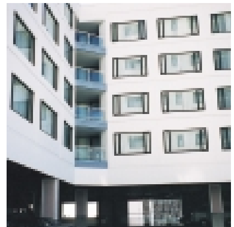
The completed Centra Hotel extension.
