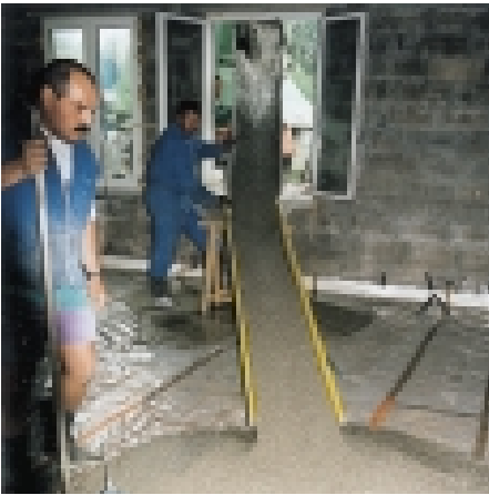
Faster placing of concrete
