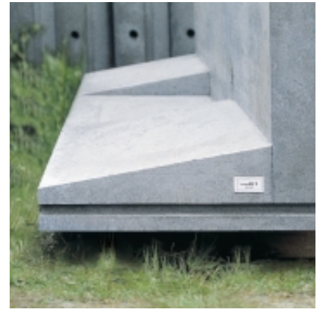
Better finish around details and edges using SCC.
