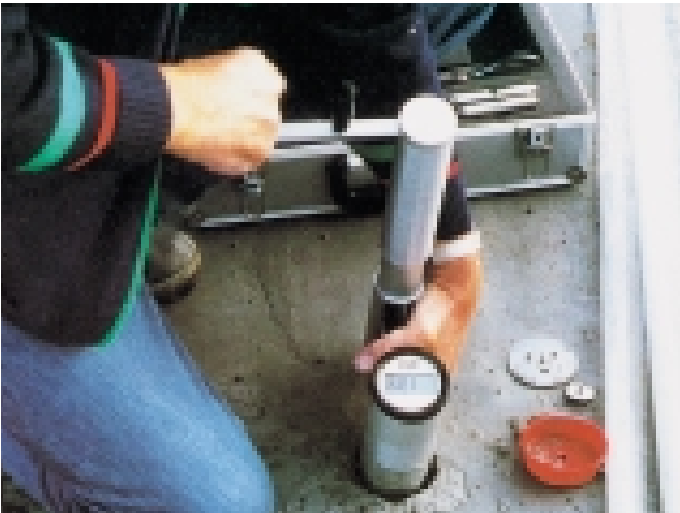
Lok-test jack in position
