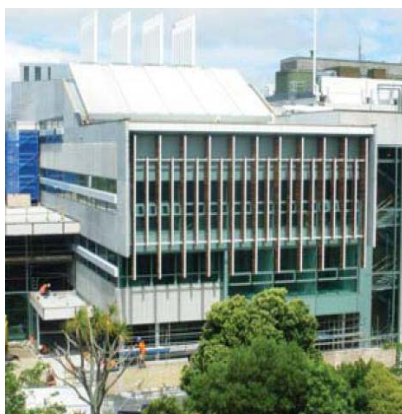
Alan MacDiarmid Building
