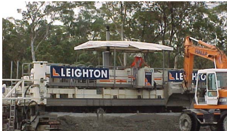
Contractors at work on a concrete road in Australia.
