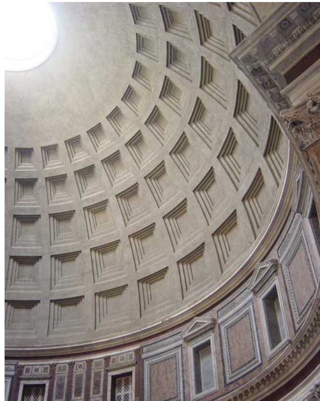
The unreinforced concrete dome of the Pantheon, Rome.
