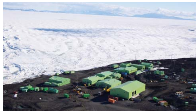
Aerial photo of Scott Base (Hillary Field Centre in the bottom right).
