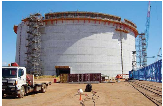
Darwin LNG tank near completion.
