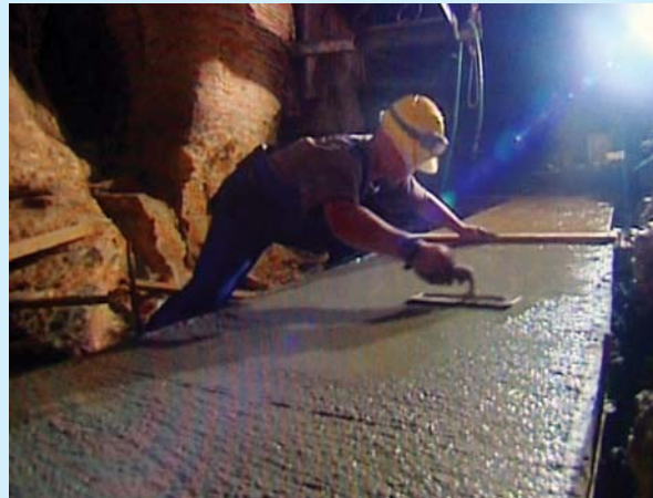
Laying the concrete paths within Ruakuri Cave.
