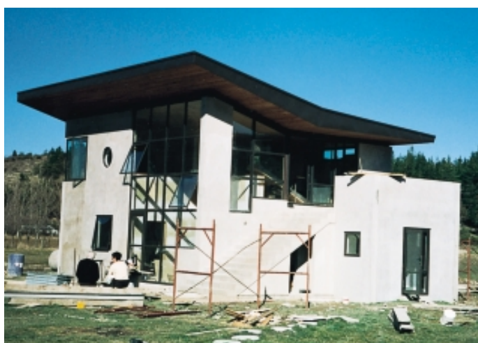
Building nearing completion.
