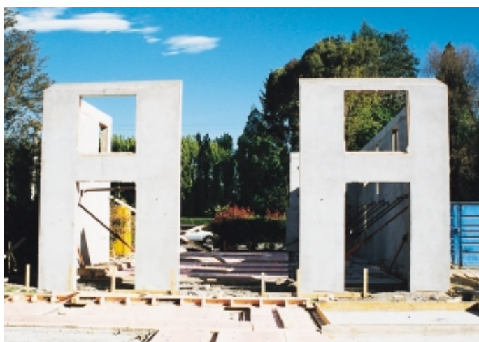
Insulated concrete panels in position and temporarily propped.
