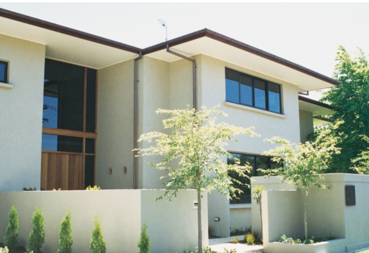
Insulated concrete panel building in Christchurch.
