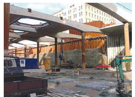
...with temporary retaining (background & secant piles to right)
