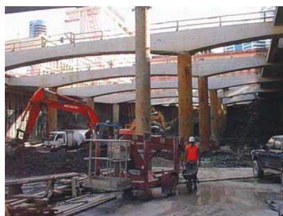
Britomart Station Roof Beams
