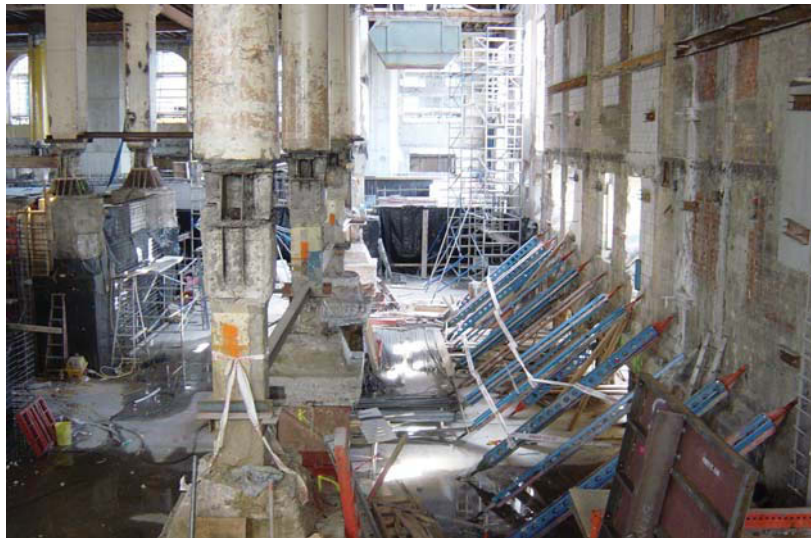
Chief Post Office alterations & strengthening showing ground floor removed and basement floor lowered.
