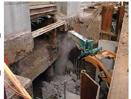
Constructing the tunnel under the front steps...
