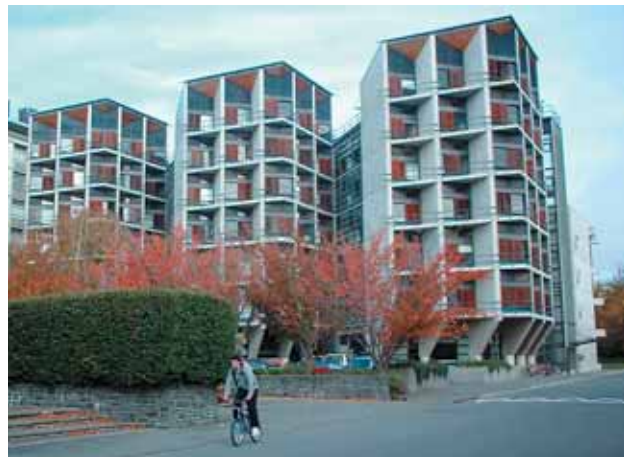
An example of high mass construction - the Maths and Science Building at Canterbury University.
