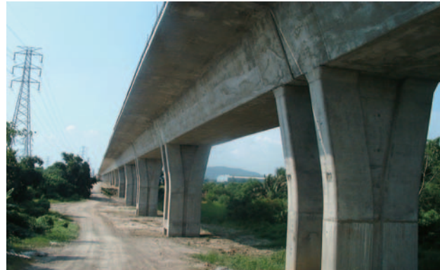
The project includes 251 kms of concrete viaducts.
