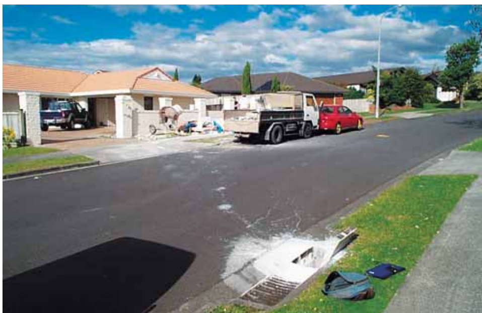
Concrete run-off - the danger to stormwater drains.
