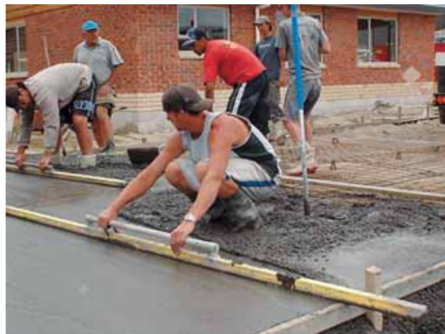
Workplace training in action - Travis from Angus McMillan Concrete Limited.
