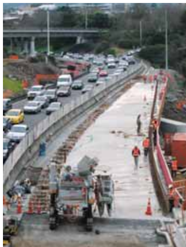
Construction underway on Auckland's spaghetti junction.
