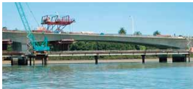
First concrete closure pour for Upper Harbour Bridge now complete.
