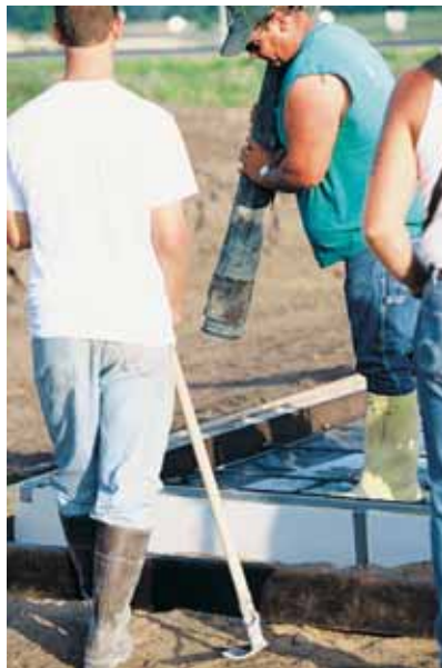
Practical applications of concrete in training. Photo: © PCA.
