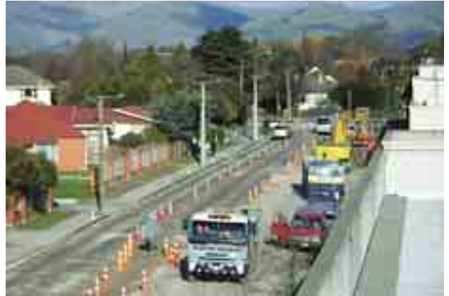
Golf Links Road, New Zealand's first recycled road in development.
