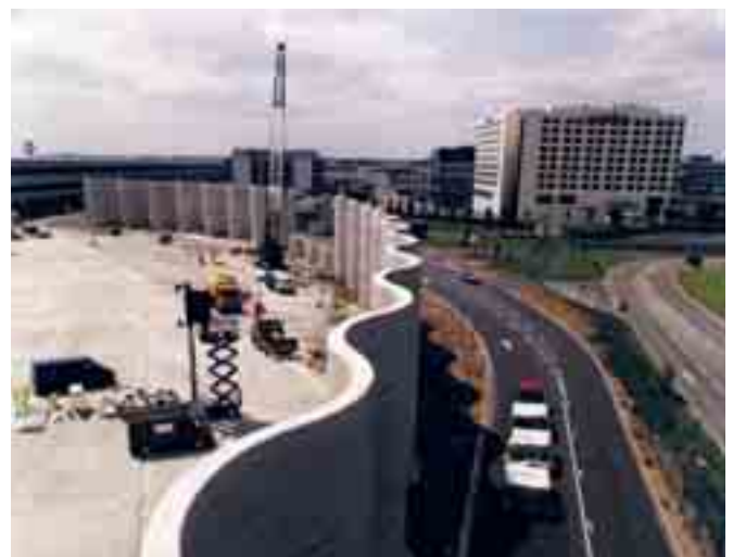
Concrete Acoustic Barrier - Wave Wall.
