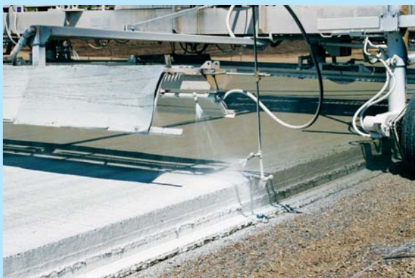
Process of curing concrete. Image courtesy of Portland Cement Association (PCA).
