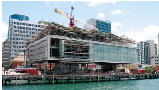
The Kumutoto Site 7 building on Wellington's waterfront under construction.
