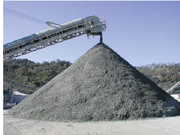
Production of Hydrated Cement Treated Crushed Rock Base (HCTCRB) in Western Australia.
