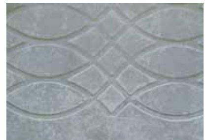
Finished precast concrete panel.
