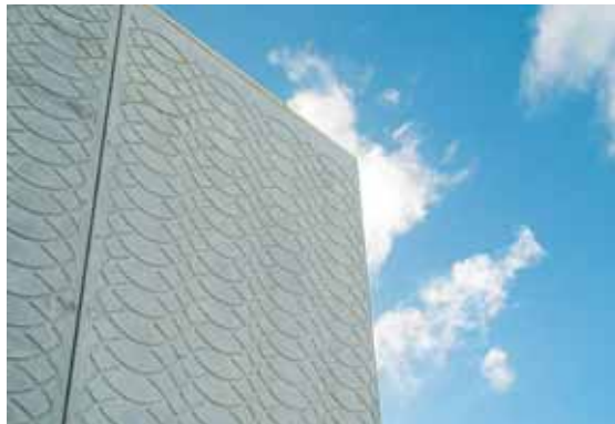
The Sanctuary's 7 m high precast concrete panels.
