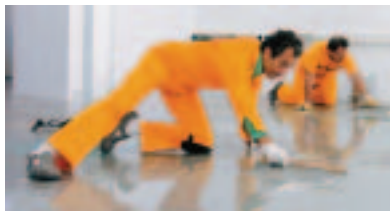
The SikaFloorSystem being applied. Image courtesy of Sika NZ Ltd.
