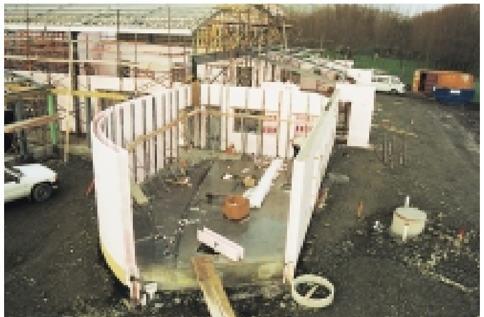
Above: Curved walls can be achieved using ICF. Below: Aerial view of church.
