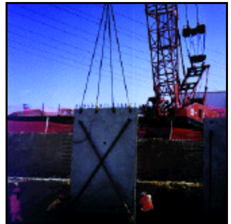
Right: Craning an 11 tonne precast wall panel into place for the MLE tank.
