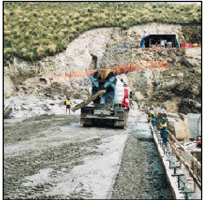
Air entrained conventional concrete is placed against D/Sshutters.
