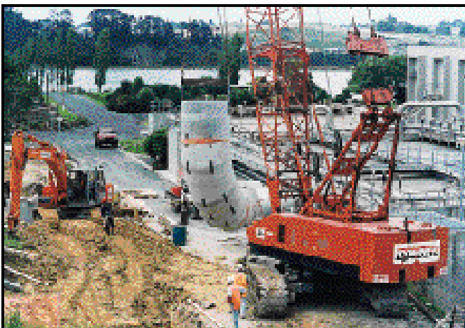
From the top: Wall panels erected for clarifier tank.
