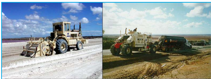
Figure 6: Insitu Stabilisation (Austrads 2006).
